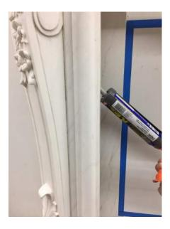
4. Apply a dot of adhesive to the top of side return edge.
