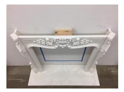
7. Double check measurements, ensuring everything is centered and the profile is aligned. Secure legs in place with adhesive/thin-set along the inner edges.
